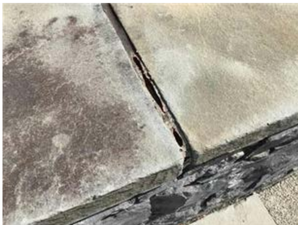
Failed sealant
